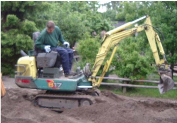
Removal of topsoil
