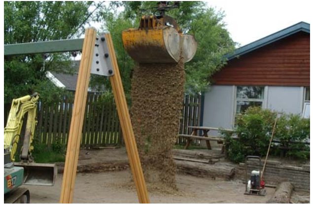
Add the subbase material
