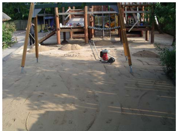
Add, if necessary, a thin layer of compactable leveling sand or crushed rock powder and compact and level it.
