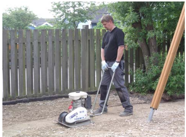
Compact the subbase
