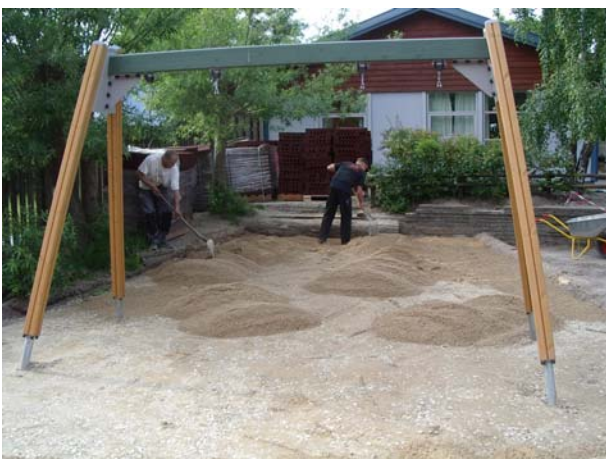
Add, if necessary, a thin layer of compactable leveling sand or crushed rock powder and compact and level it.
