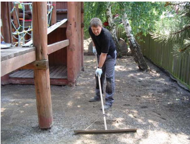
Level out the subbase material
